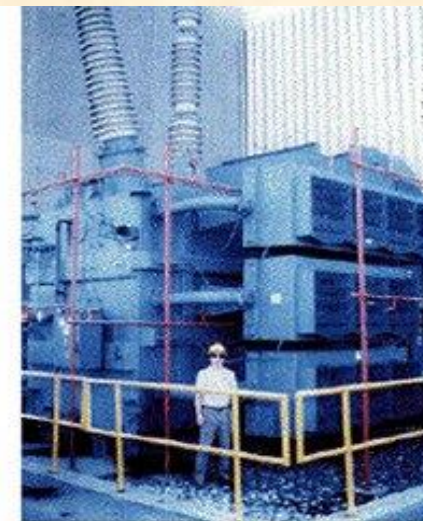
PJM Public Service Step Up Transformer Severe internal damage caused by the space storm of 13 March, 1989
